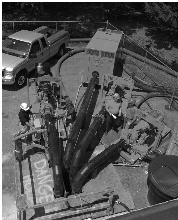
The pumps were staged in an area only 30 by 30 feet.
